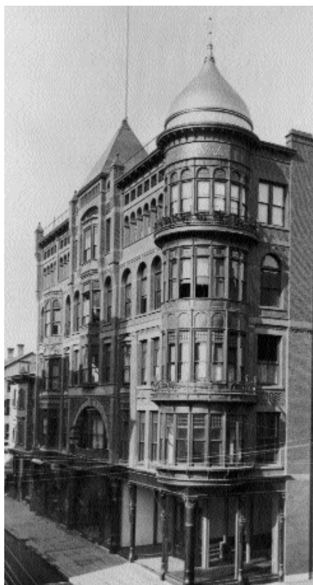
Photo of Conrad Building c. 1890, courtesy of the Rhode Island Historical Society.
